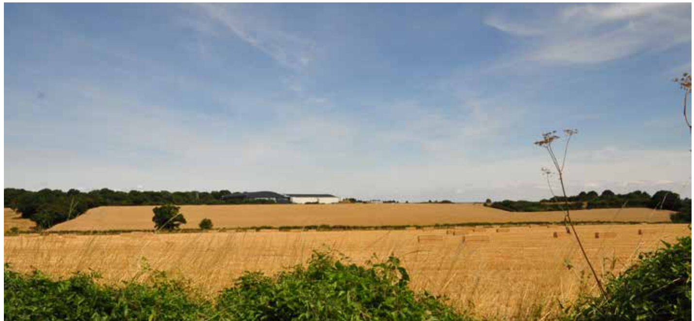
Figure 82: Dyson repurposing of aircraft hangar for R+D use at RAF Hullavington
