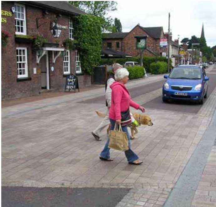
Figure 24: Example of a street in Poynton, Cheshire where the use of materials and vertical deflection, provide a pedestrian priority environment
