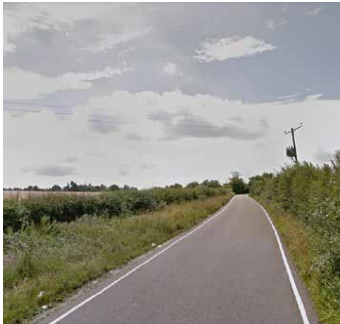
Figure 7: Rye Hill Road looking south
